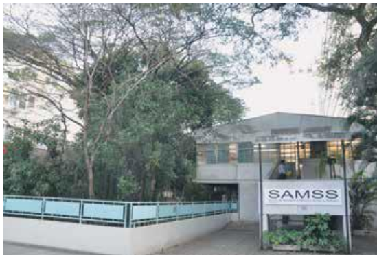
The former SAMSS building next to the HCFMUSP Administration Building will be renovated to host offices for clinical research
