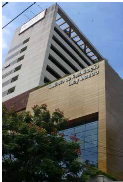
Headquarters of Lucy Montoro Rehabilitation Institute, in Santo Amaro
