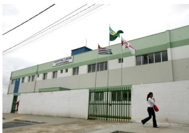
Front view of the Local Hospital of Sapopemba
