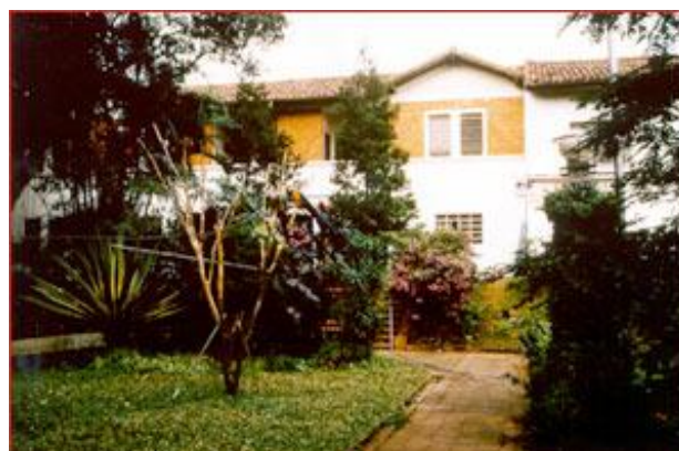
internal garden of Auxiliary Hospital of Cotoxó
