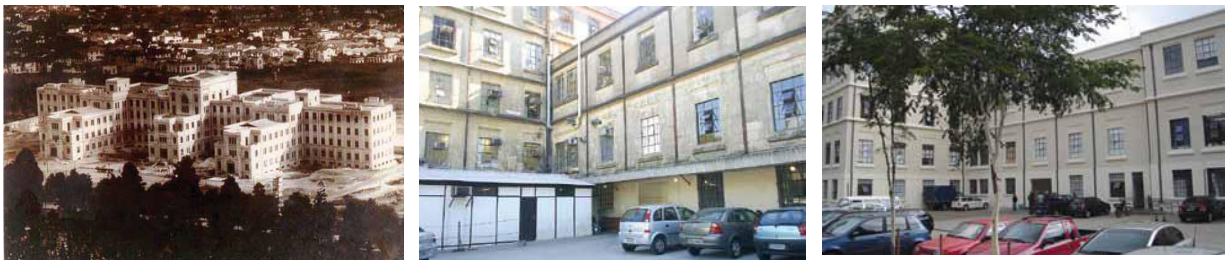
Project of Restoration and Modernization of FMUSP, coordinated by FFM from 2000 to 2008 – Sequence of images of the headquarter building of FMUSP: on the left the building in 1931 right after being opened; in the middle, the back side of it before the reform; on the right the building after the reform.
