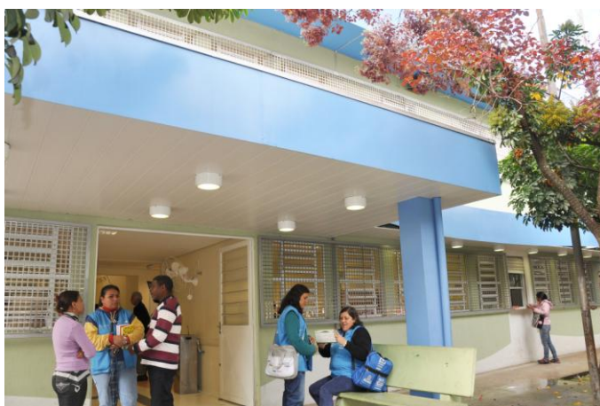
Front view of UBS - Vila Dalva
