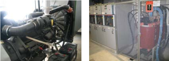
Transforming Cabins after restoration
