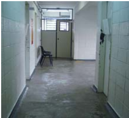
1 st floor aisle from Vila Dalva UBS before restoration
