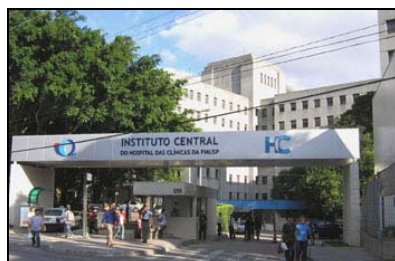
ICHC Central Building
