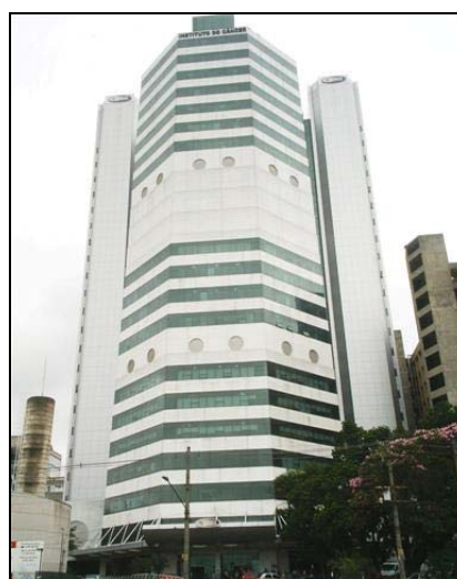
Front of ICESP Building
