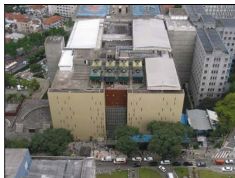
Ambulatory Building Area
